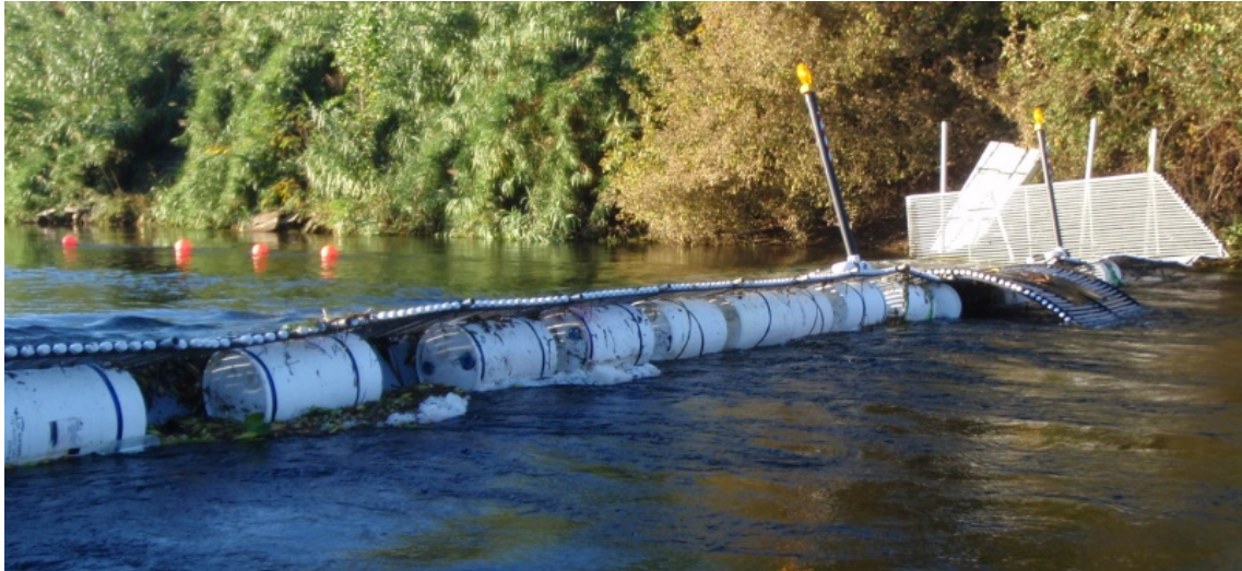
Figure 2. Photograph of the flotation barrels lining the underneath of the resistance weir.
